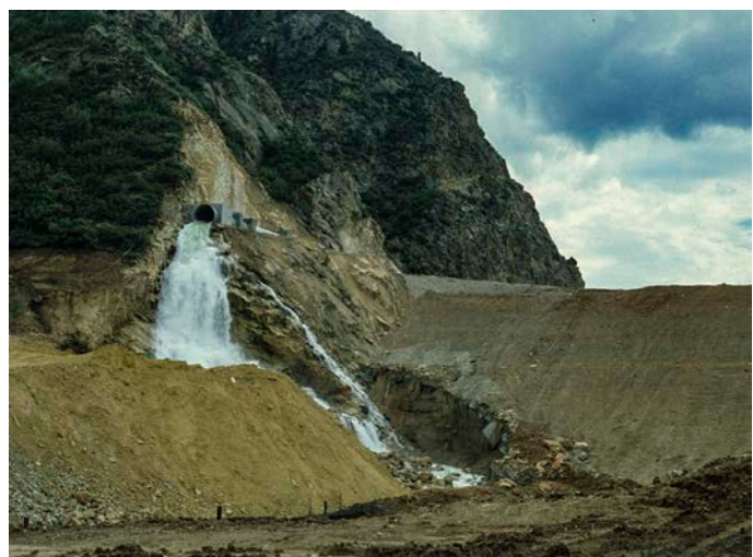
Water from the new overflow pipe cascades down a bedrock spur, safely away from the front of the landslide dam.
