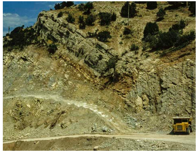
The two limestone units exposed in the Billies Mountain road cutting; the strong upper bed forms a natural scarp, but the weak lower bed is having to be cut back and terraced.
