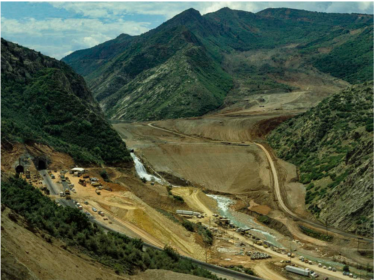
The landslide and dam seen from the new road on Billies Mountain, with the lake extending away to the left.
